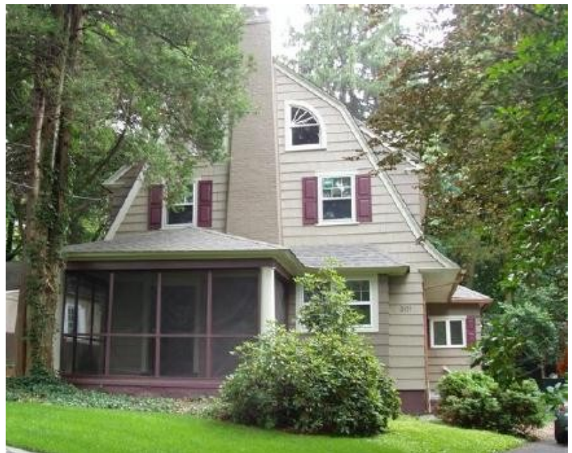
The Dutch Colonial featured a gambrel roof and curved eaves
